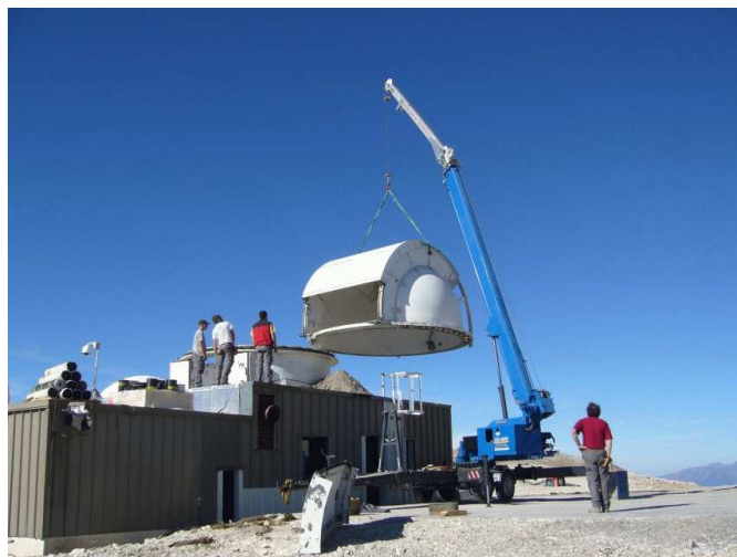
Figure 6: Dismounting of the POM2 astrodome.
